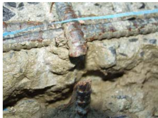
Fig. 1 Fractured stirrup
