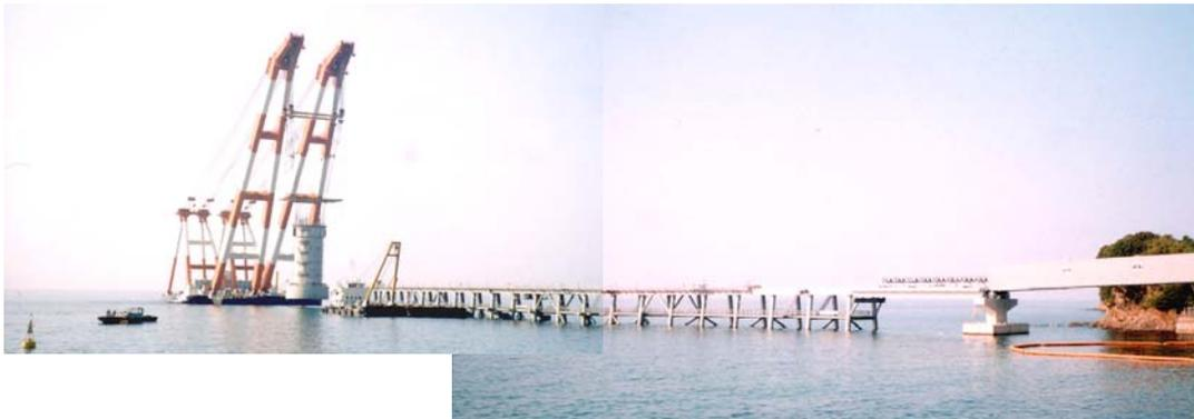
**Photo1** View of protection just before skirt penetration
