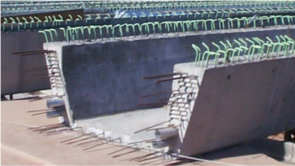
Fig. 1 NDOT Precast U-Girder for McCarran/US395 Bridge
