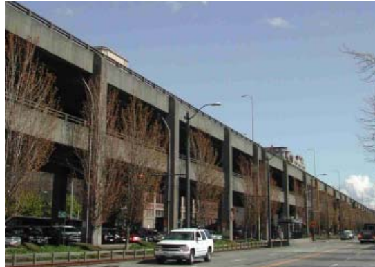
Figure 1, The Alaskan Way Viaduct
