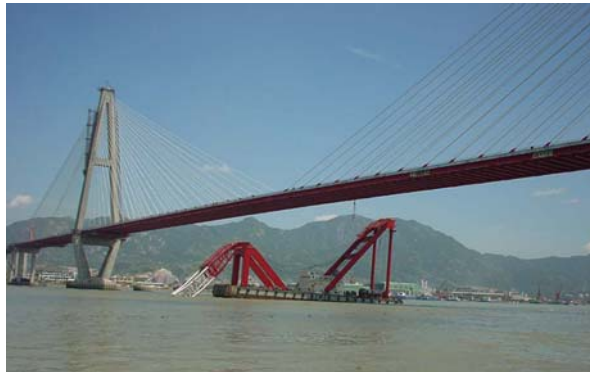
Barge Impact to Stay Cables, Fuzhou, China
