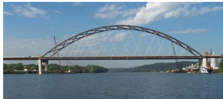
Blennerhassett Island Network Tied Arch
