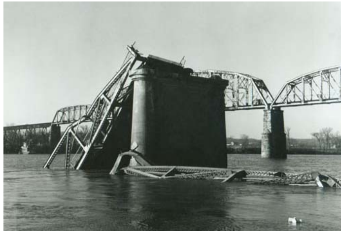
Silver Bridge Collapse – December 15, 1967
