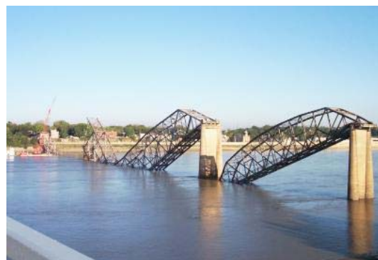
Cape Girardeau Truss Demolition
