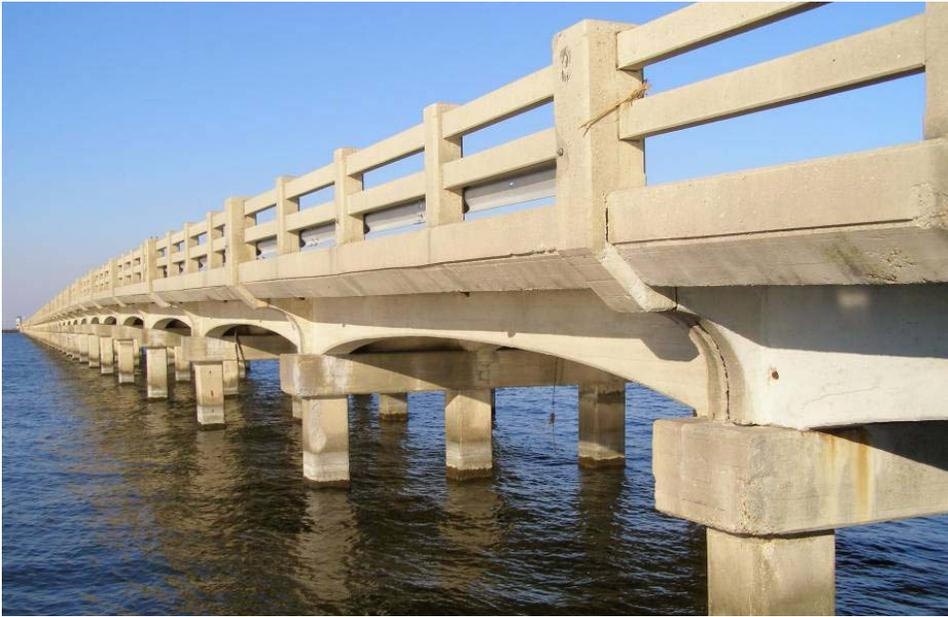
Figure 3. Cast-in-Place Concrete US-11 Bridge over Lake Pontchartrain (photo credit: J. O'Connor, MCEER).
