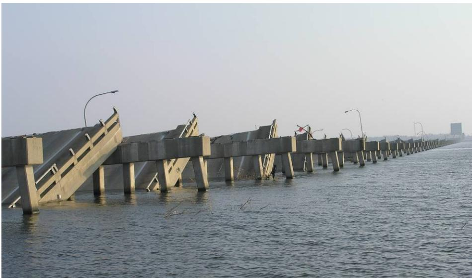
Figure 2. US-90 Biloxi-Ocean Springs Highway Bridge with Superstructure Spans Displaced North Off Their Piers (photo credit: J. O'Connor, MCEER).
