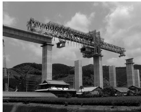
*Photo 5-1: Overhead launching truss*
