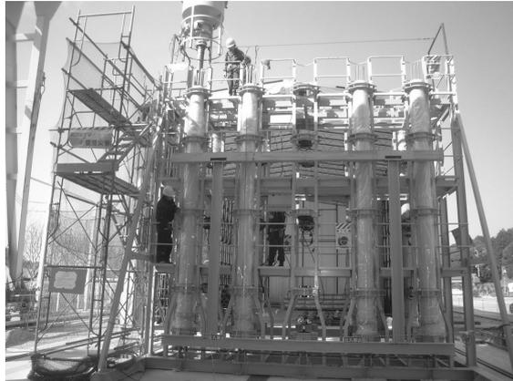
*Photo 6-3: Prefabrication of strut*
