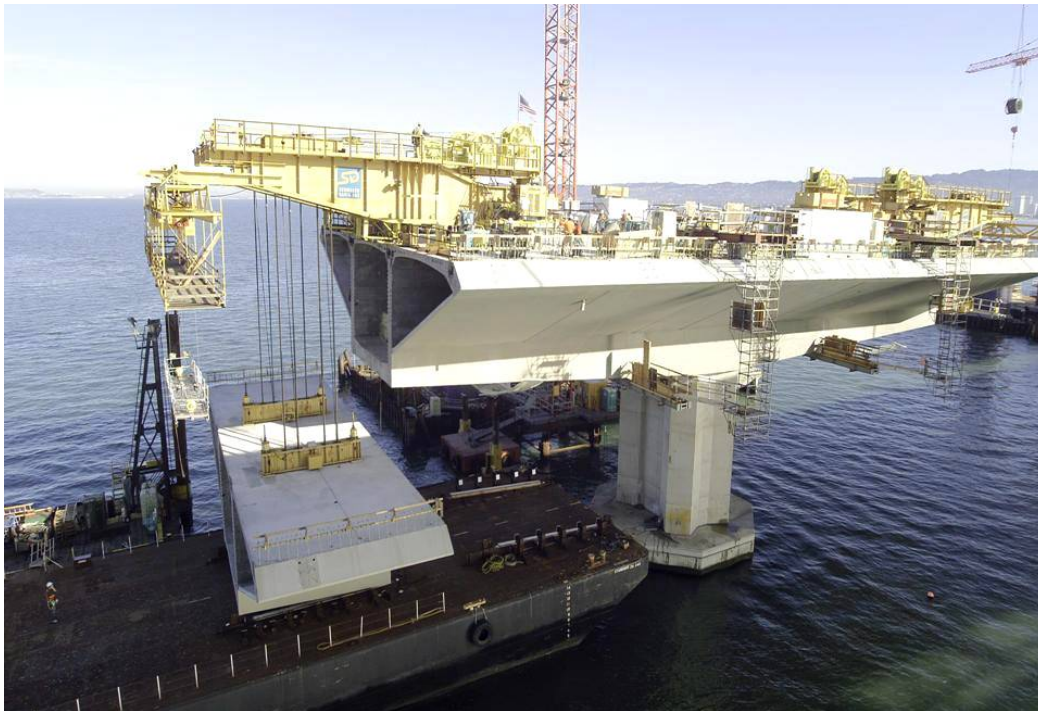
FIGURE 10: LIFTING CONCRETE SEGMENTS INTO PLACE
