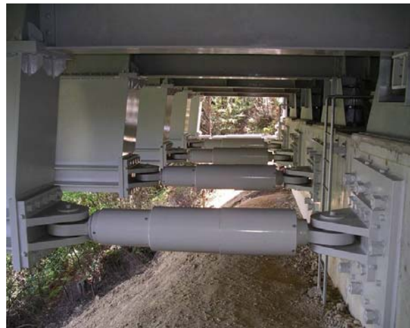
Photo 1 DAMPERS INSTALL (4A)
