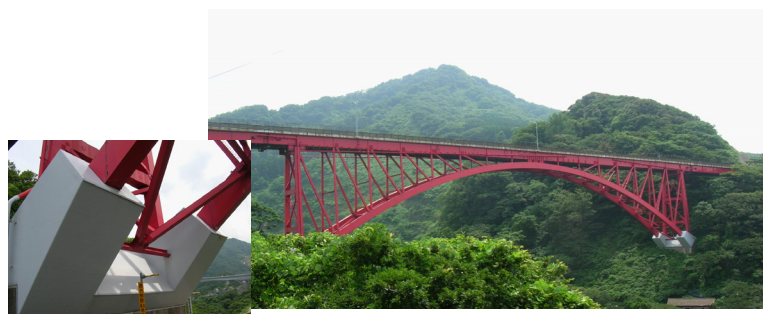
Photo 3 A long span bridge that did not suffer damage during the 2007 Niigata-ken Chuetsu-oki earthquake (Mj6.8) because of seismic reinforcement provided by the PWRI.
