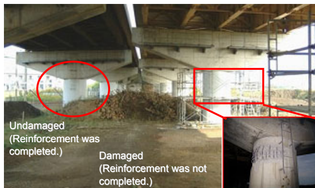
Photo 2 Undamaged and damaged piers next to each other following the 2004 Niigata Chuetsu earthquake (Mj6.8), in which undamaged piers were reinforced as part of a seismic reinforcement program
