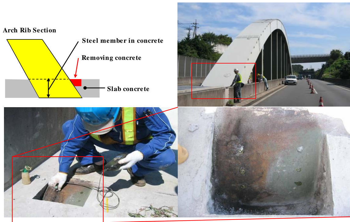
Fig.11 Inspection of steel member in concrete at bridge of NEXCO (Mono arch Lohse bridge)
