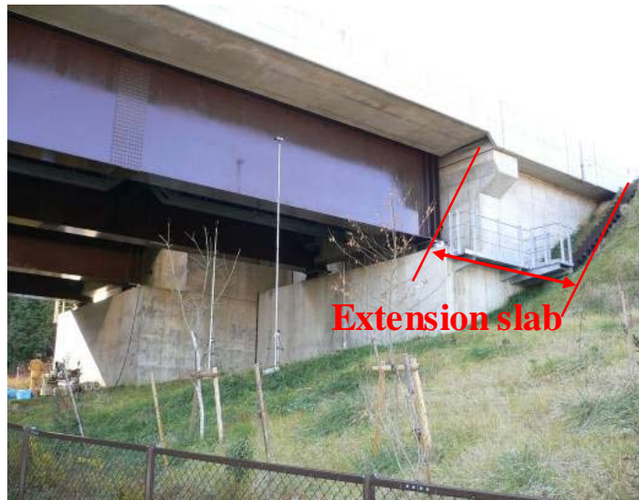
Fig.10 Extension slab system at Bridge of NEXCO
