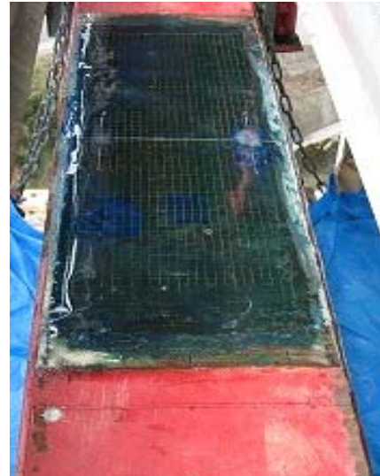
fig.13 Repair by carbon fiber sheets at Asarigawa bridge of Chuo expressway
