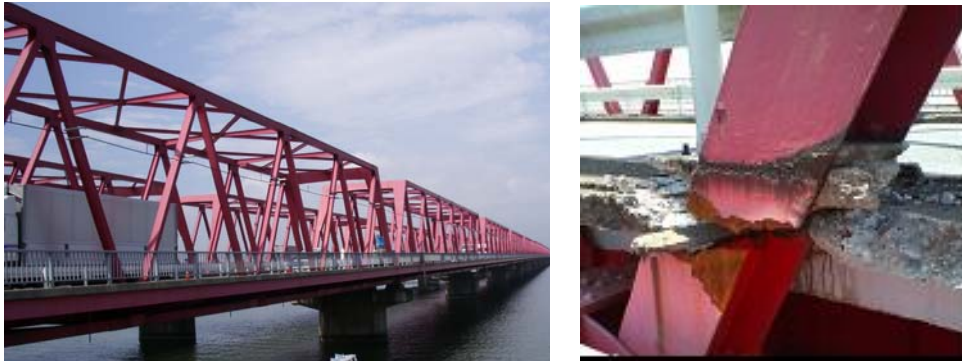
Figure2 Failure of diagonal member of truss bridge
