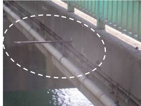
Figure5 Corrosion of prestressing steels 3) Figure6 Falling out of prestressing steel
