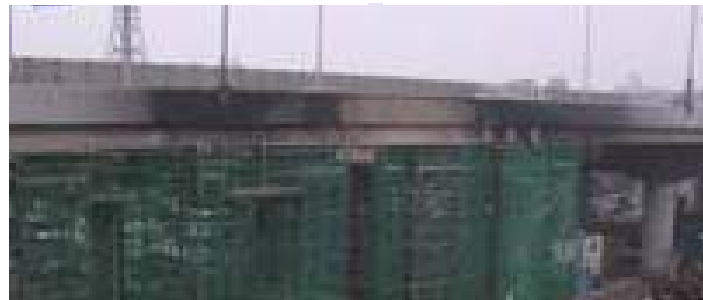
Figure7 PC beam suffered from fire
