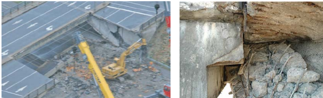
Figure2 Failure of diagonal member of truss bridge
