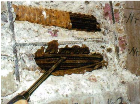
Figure5 Corrosion of prestressing steels 3) Figure6 Falling out of prestressing steel
