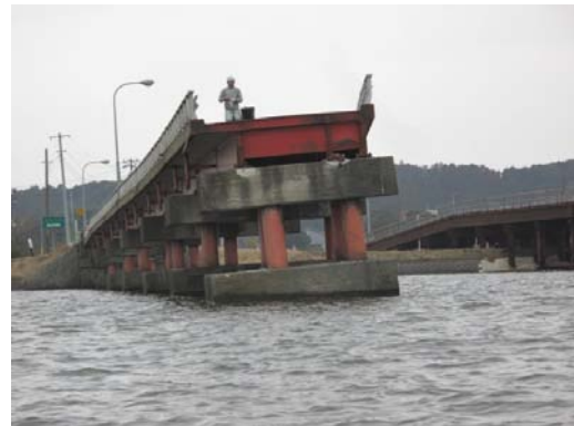
Photo 4 Collapse of Steel Pile-bent Columns
