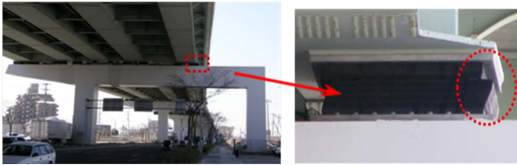
Photo 5 Rupture of Elastomeric Rubber Bearings in Sendai Tobu Viaduct (P54, Two-column Steel Frame)
