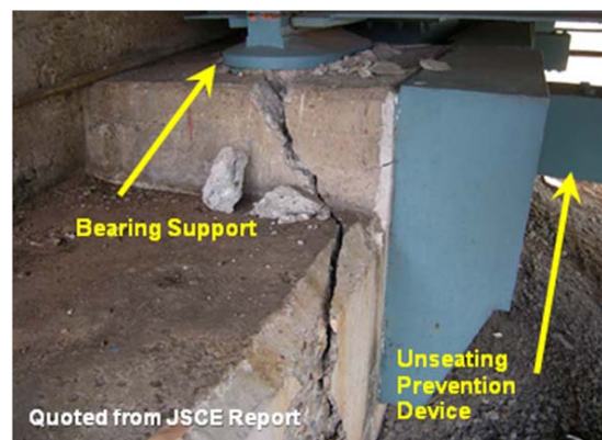
Photo 9 Crack to Pier Top Affects Attachment
