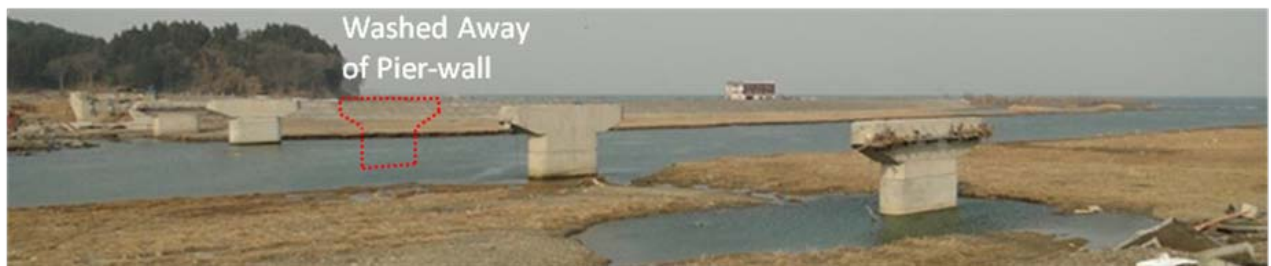
Photo 10a Washed Away of Steel Superstructure and Pier-wall (Koizumi Bridge)
