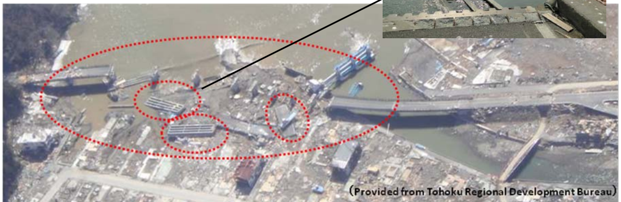
Photo 11 Washed Away of PC Superstructure (Utatsu Ohashi Bridge)
