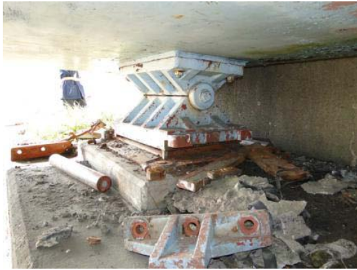
Photo 2 Damage of Steel Bearing Support
