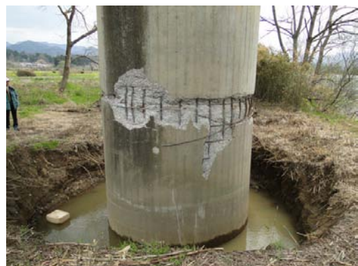
Photo 1 Damage of Reinforced Concrete Columns at Cut-off Section of Longitudinal Reinforcement
