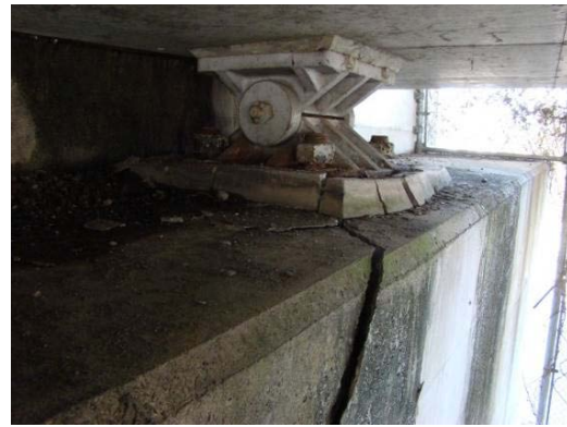
Photo 3a Damage of Pier Top
