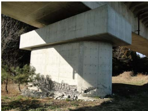
Photo 1 Damage of Reinforced Concrete Columns at Cut-off Section of Longitudinal Reinforcement
