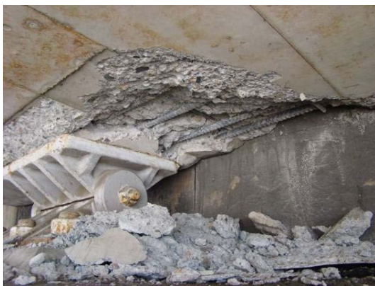
Photo 3b Damage of Attachment of Bearings to Superstructure
