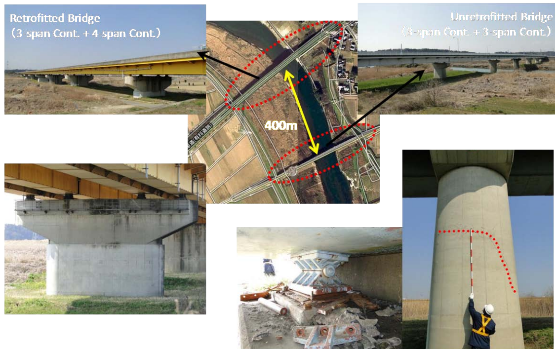
Photo 7 Comparison of Seismic Performance between Adjacent Two Bridges (Nakagawa Bridge and Kunita Ohashi Bridge)
