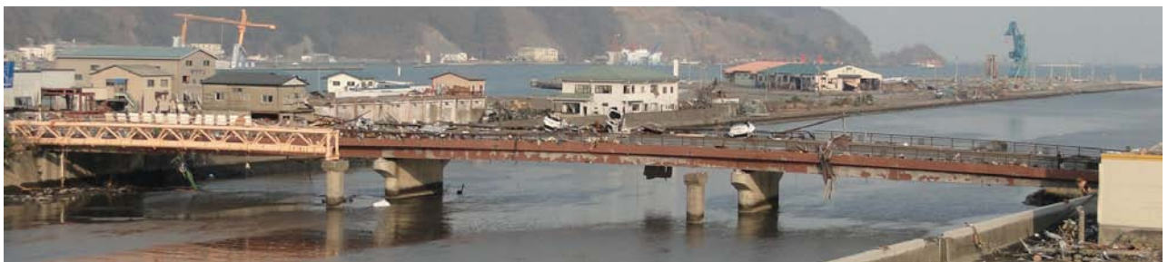
Photo 12 Bridge Survived Washed Away Due to Tsunami (Yanoura Bridge)
