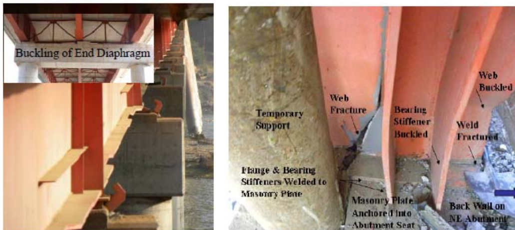
(a) Girder offset and cross frame buckling (b) Girder fracture at the north abutment
