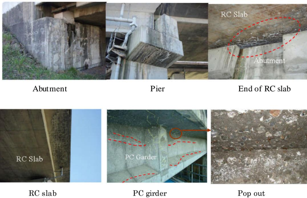
Fig.6 Cases of ASR deterioration
