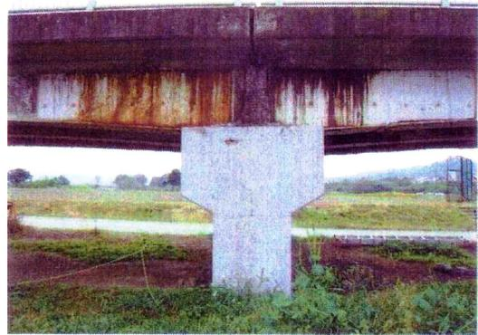
Fig. 2 Steel plates bonded on the webs of concrete girders
