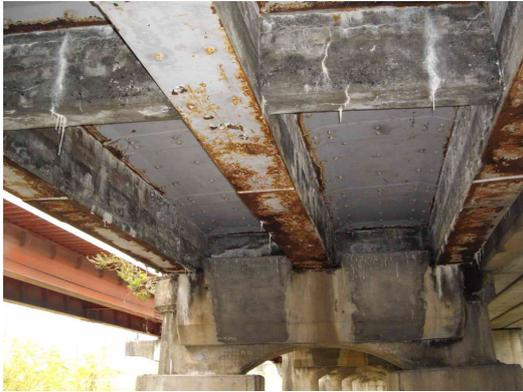
Fig. 1 Steel plates bonded to the soffit of decks and girders in a concrete bridge
