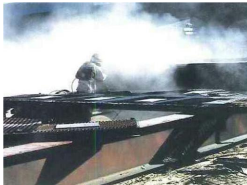
Fig.7 Cleanliness processing by blasting(According to ISO 8500-1 Sa2.5)
