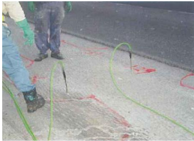
Fig.10 Shows resin being injected
