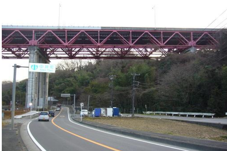
Fig.8 The bridge repaired by overlaying floor slab
