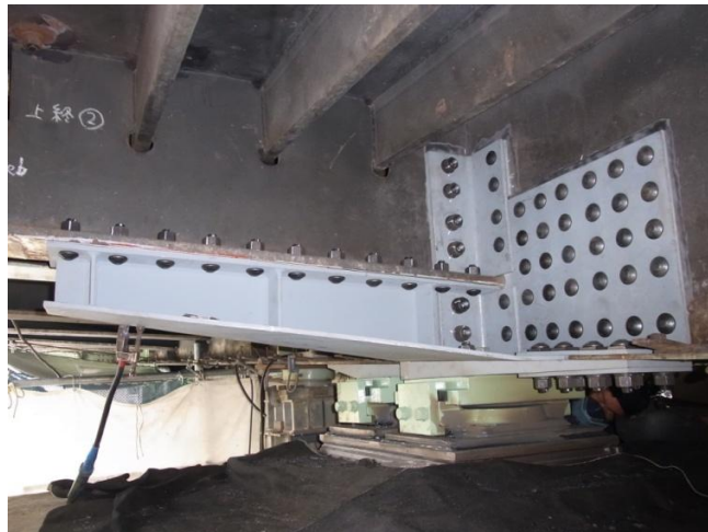
PHOTO 4 GIRDER G7 AT THE COMPLETION OF EMERGENCY REPAIR
