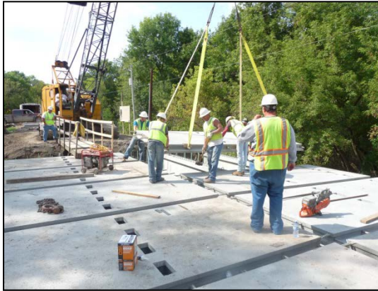
(a) Placing of waffle deck panels
