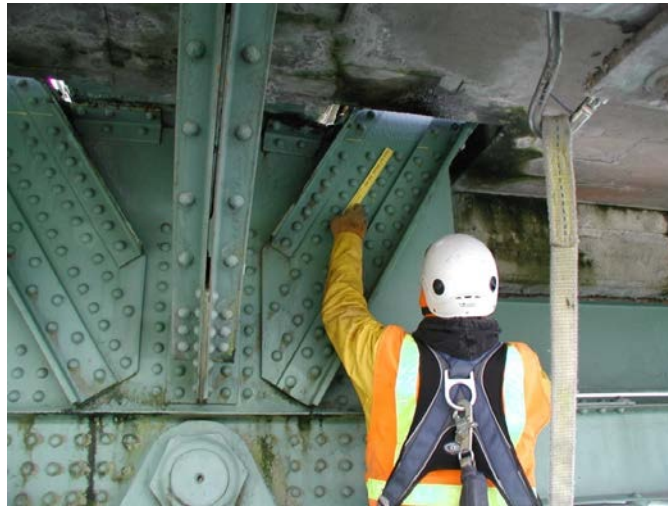
FIGURE 1 – EXAMPLE OF STATE-OF-THE-PRACTICE METHOD USED TO COLLECT FIELD DATA ON GUSSET PLATE CONNECTION GEOMETRY
