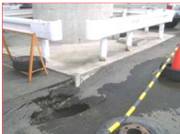
D-6 Ground Fissures, Pavement Collapse (Level 5)
