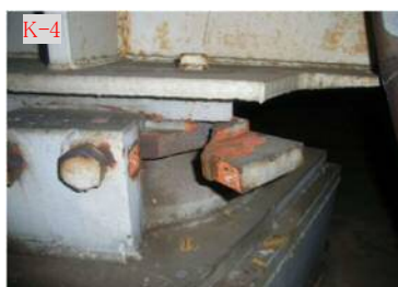
Figure 5-9 (center) Crack of Upper Bearing
