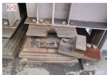
Figure 5-8 (left) Fractured Bolts
