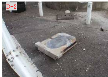
Figure 5-1 (left) Missing Upper Bearing Figure 5-2 (center) Fallen Upper Bearing Figure 5-3 (right) Missing Displacement Limiter
