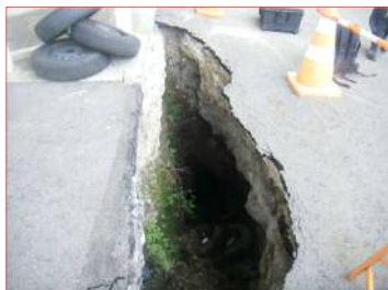
D-6 Ground Fissures, Pavement Collapse (Level 5)
