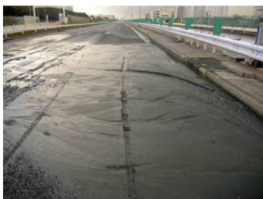
Figure 4-4 (left) Pavement Damage due to Liquefaction Figure 4-5 (center) Missing Bridge Bearings Figure 4-6 (right) Truss Component Damage
