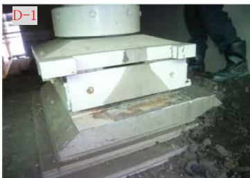
Figure 5-4 (left) Fallen Displacement Limiter Figure 5-5 (center) Missing Side Block Figure 5-6 (right) Fallen Side Block
