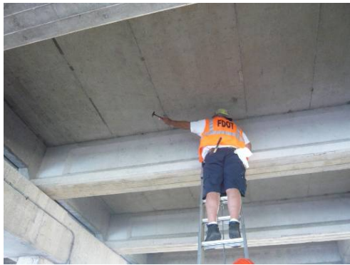
FIG. 16: HAMMER SOUNDING BY FDOT CERTIFIED BRIDGE INSPECTOR
