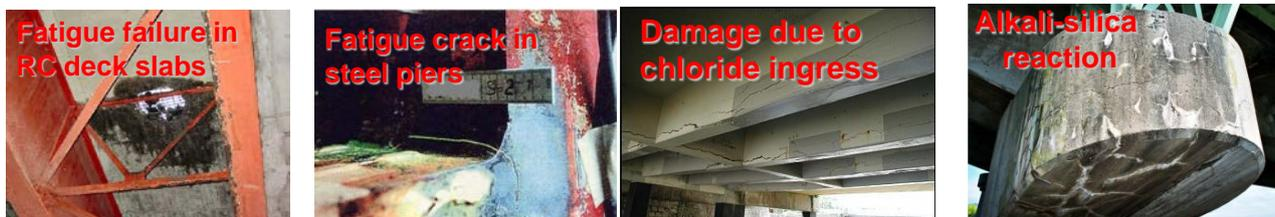
Fig. 1 Examples of damage
