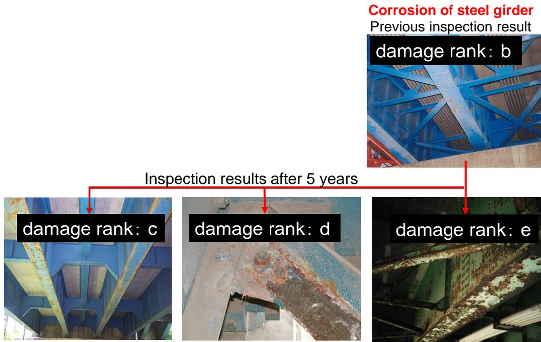
Fig. 6 Example of inspection results relating to the corrosion of a steel girder bridge
