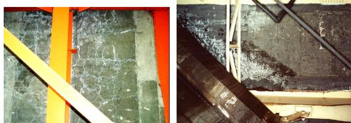
Fig. 11 Example of cracks in the deck of plate girder bridges
