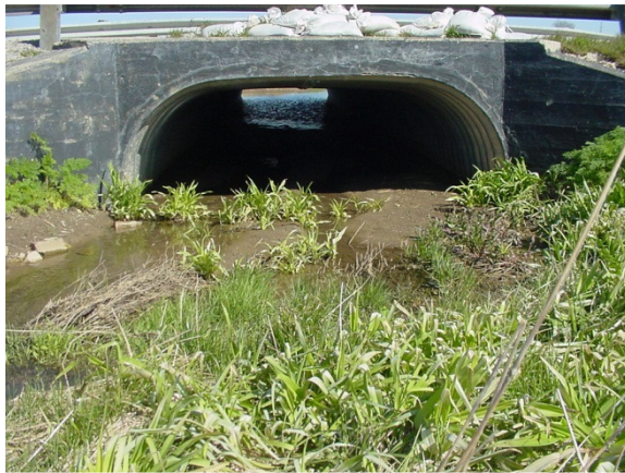
Figure 2 Structural Plate Box Culvert
