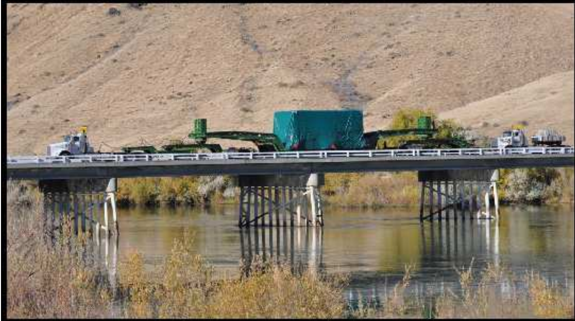
A LONG PERMIT VEHICLE DISTRIBUTING THE LOAD OVER SEVERAL SPANS
