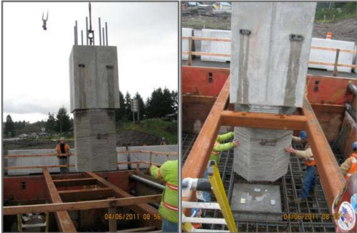
Fig. 9: Construction sequences for placement of precast column segment into footing
