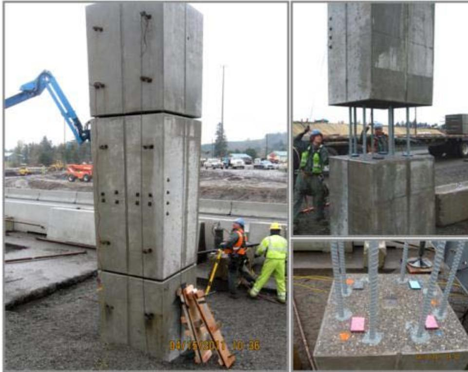
Fig. 10: Column Segment Placement
