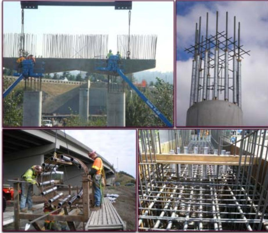
Fig. 4: Precast Bent Cap under Construction in Washington State
