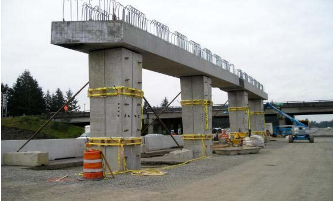
Fig. 11: Grouting the Joints between Column Segments and between Column and Bent Cap
