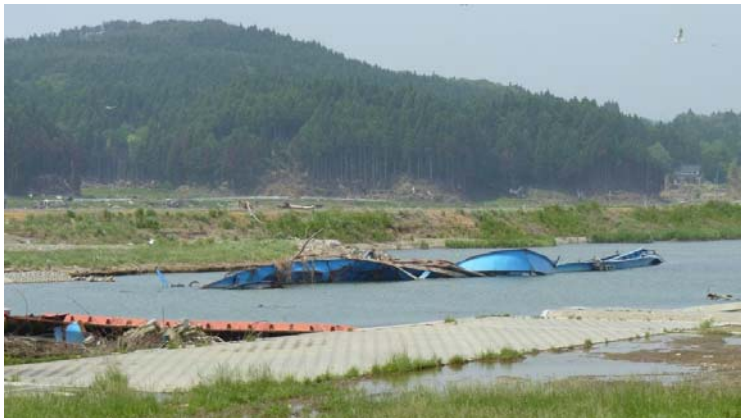
FIGURE 1. GIRDERS FROM KOIZUMI BRIDGE 400 M UPSTREAM IN TSUYA RIVER CHANNEL, TOHOKU EARTHQUAKE, 2011 (PHOTO: E. MONZON)
