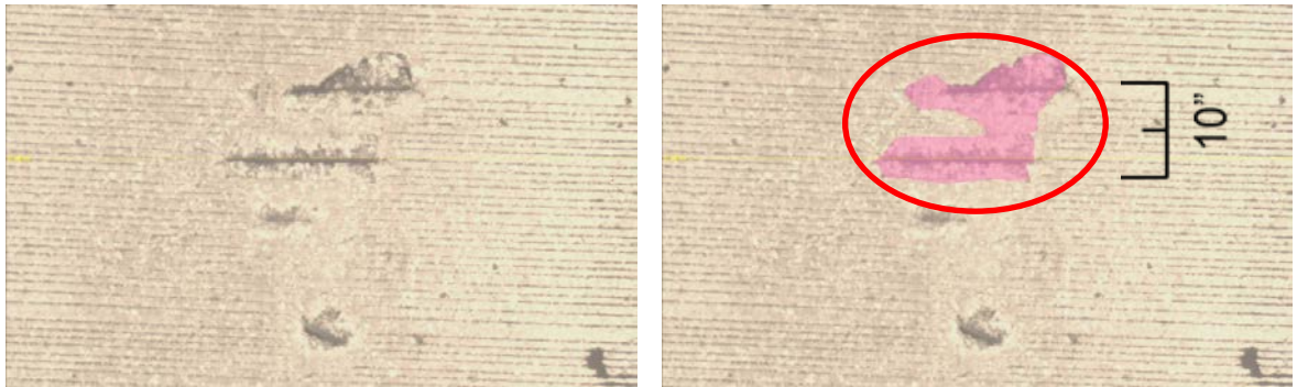
Fig.13: An Example of a Pothole with Corroded Rebar Exposed
