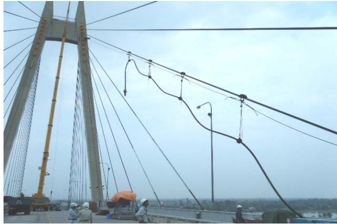
Figure 16 Installation of new stay cable
