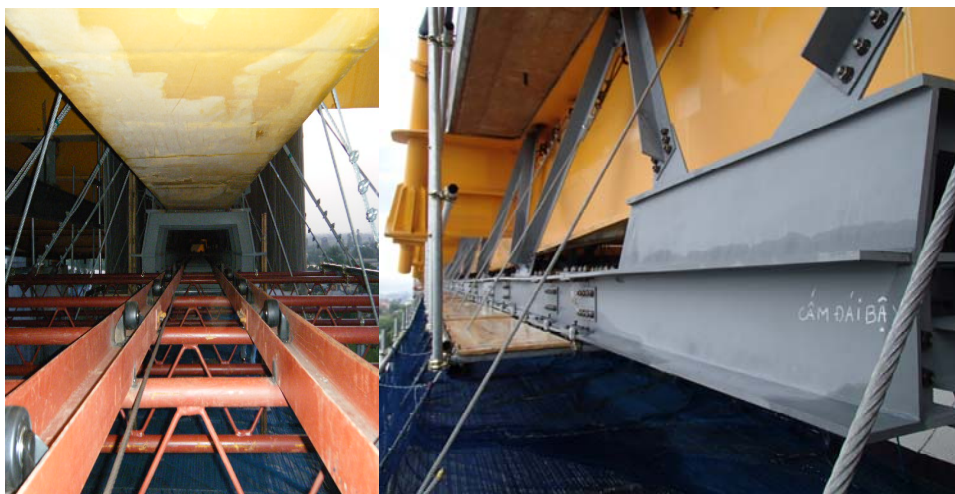
Figure 11 Temporary Bypass Truss
