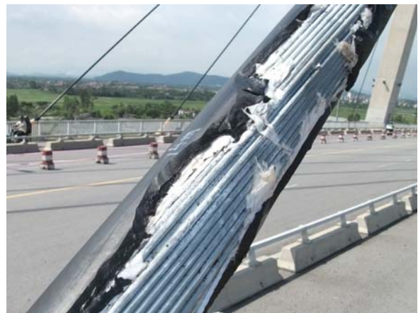
Figure 7 Cable Damage
