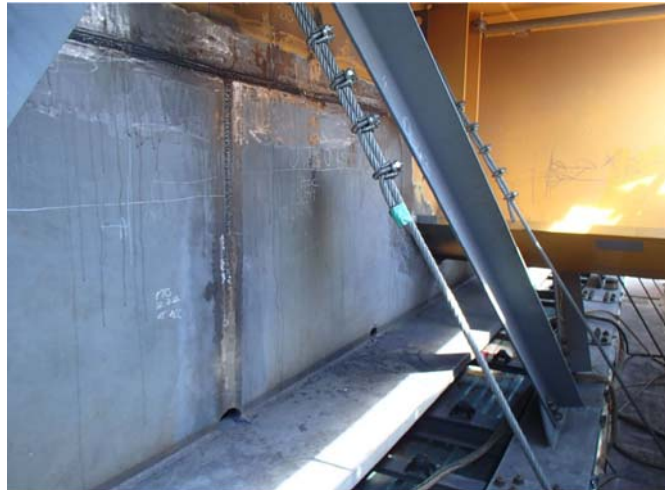
Figure 14 Installation of new parts at site
