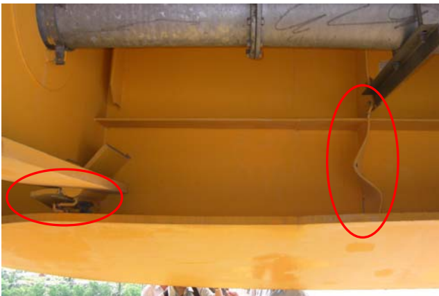
Figure 6 Buckled Stiffeners
