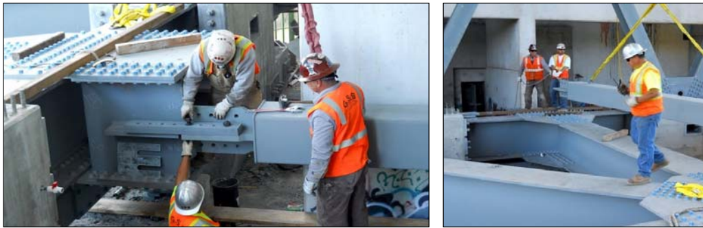
FIGURE 16. BRB INSTALLATION
