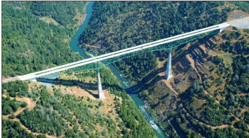
FIGURE 1. AERIAL VIEW OF FORESTHILL BRIDGE LOOKING NORTH
