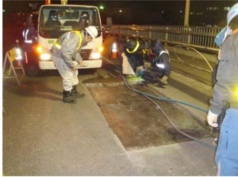
(a) Visual observation of deck surface after removal of asphalt layer
