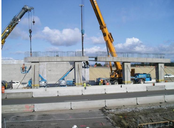
Figure 12. Placement of precast concrete cap beam.
