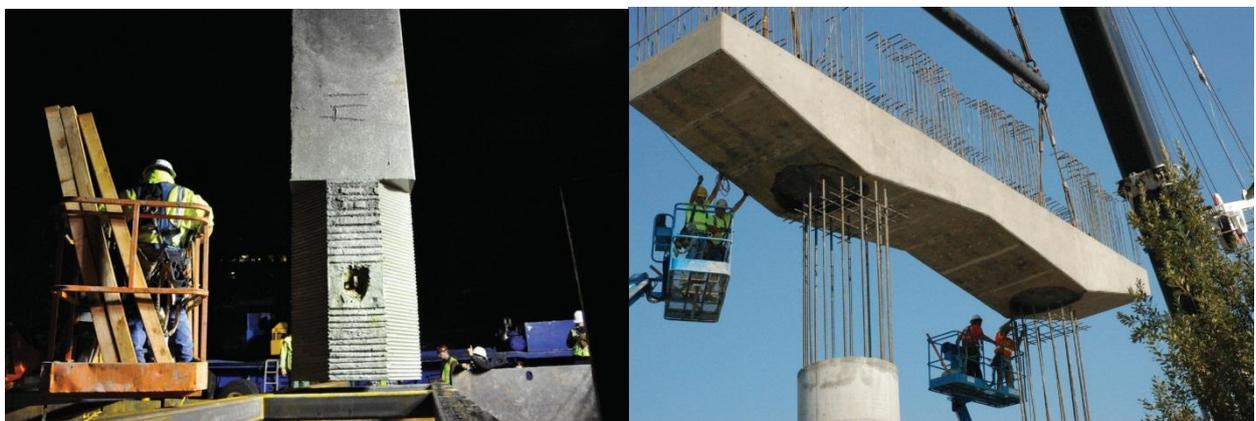
Figure 7. Previous use of precast concrete cap beam that used in Washington State.
