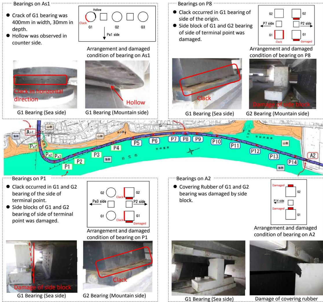
**Fig.3** Damage of Lead Rubber Bearings in Asahi viaduct
