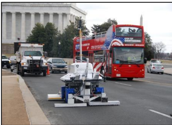
Figure 4. The RABIT™ Bridge Deck Assessment Tool on the Arlington Memorial Bridge.
