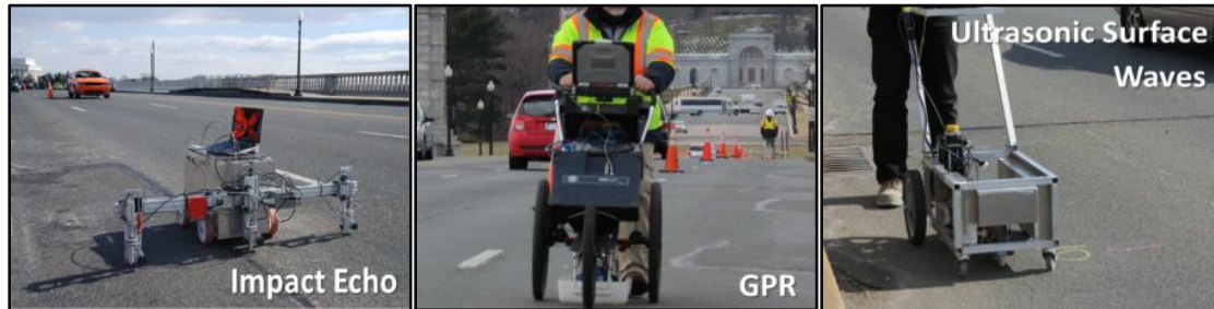
Figure 3. Manual NDE Tools used during the Arlington Memorial Bridge (AMB) Survey.
