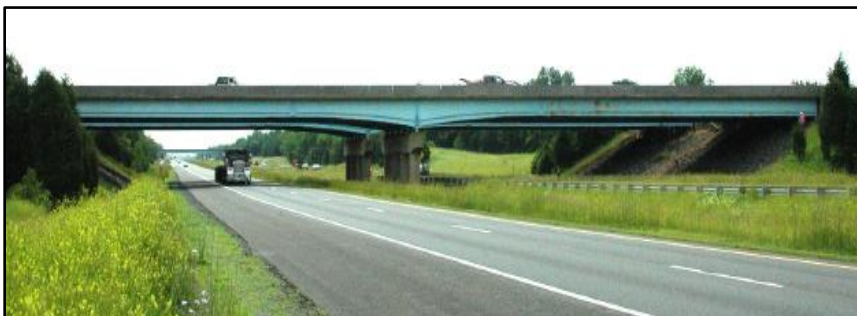
Figure 7. Overview of the Virginia Pilot Bridge in Prince William County, VA
