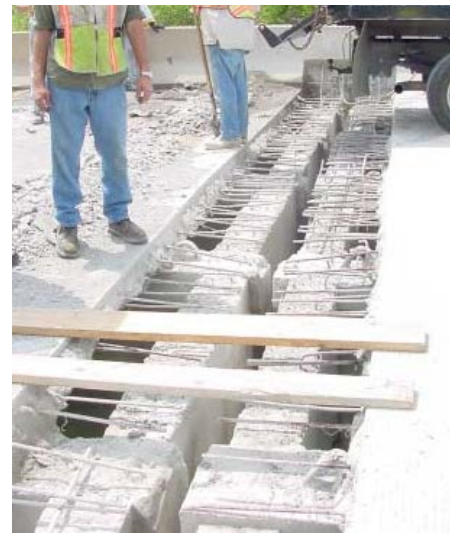
Figure 3. Typical Detail (and picture) used for Elimination of Joints in Virginia
