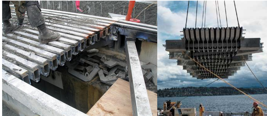
Figure 2: Expansion joint rehabilitation Project
