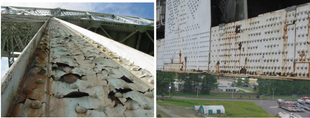
Figure 3: Condition of steel bridges and need for repainting
