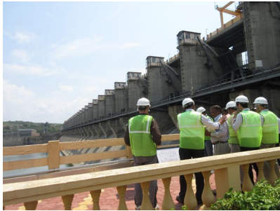
Photo 3-9 Field visit to Almatti Dam
