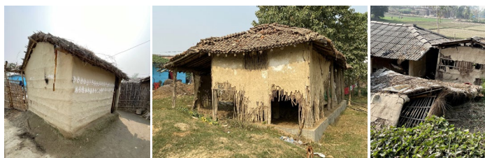
Photo 3-14 A typical MT-house (left) and damaged MT houses
