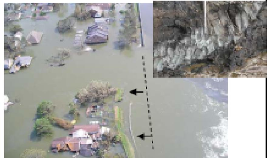
Displacement of wall and part of levee
