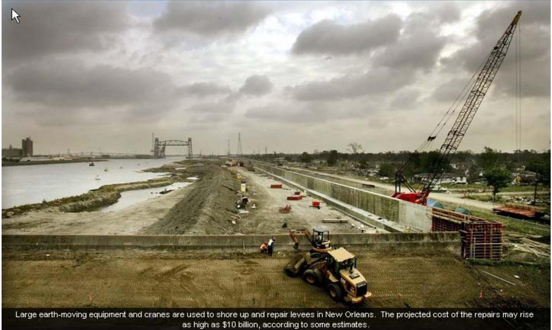
Large earth-moving equipment and cranes are used to shore up and repair levees in New Orleans. The projected cost of the repairs may rise as high as \$10 billion, according to some estimates.
