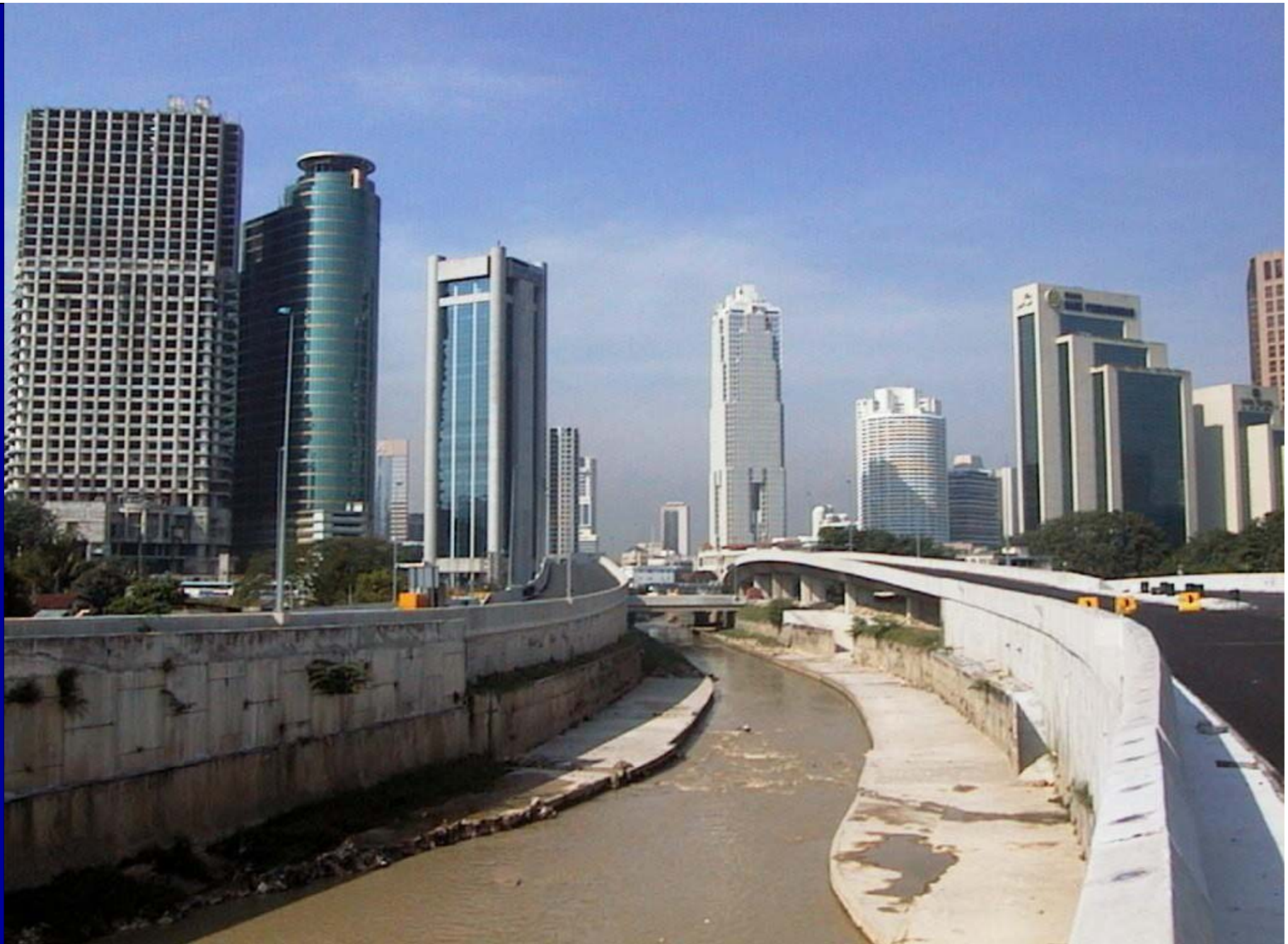
River Levees (Walls) in City Centre
