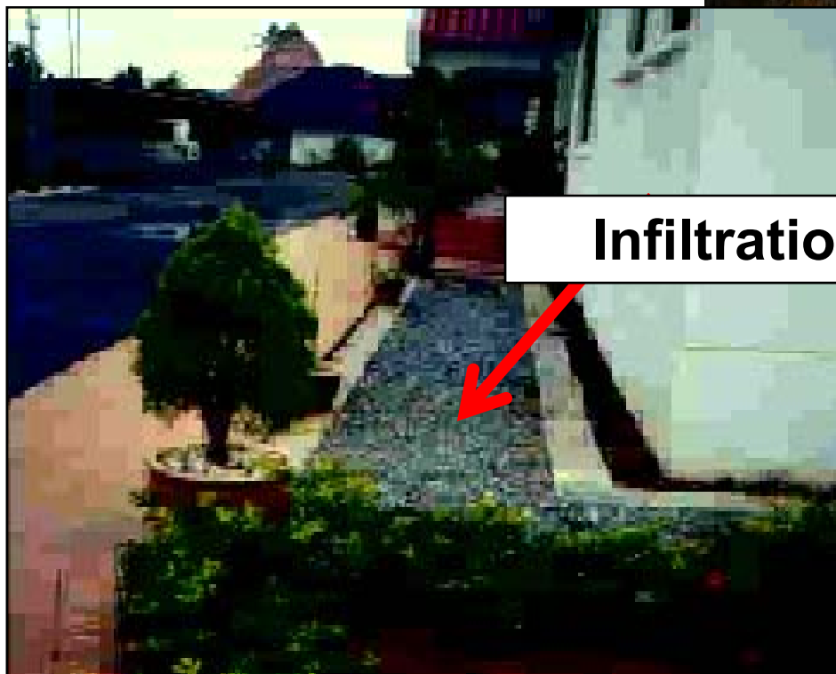
Infiltration System at housing perimeter
