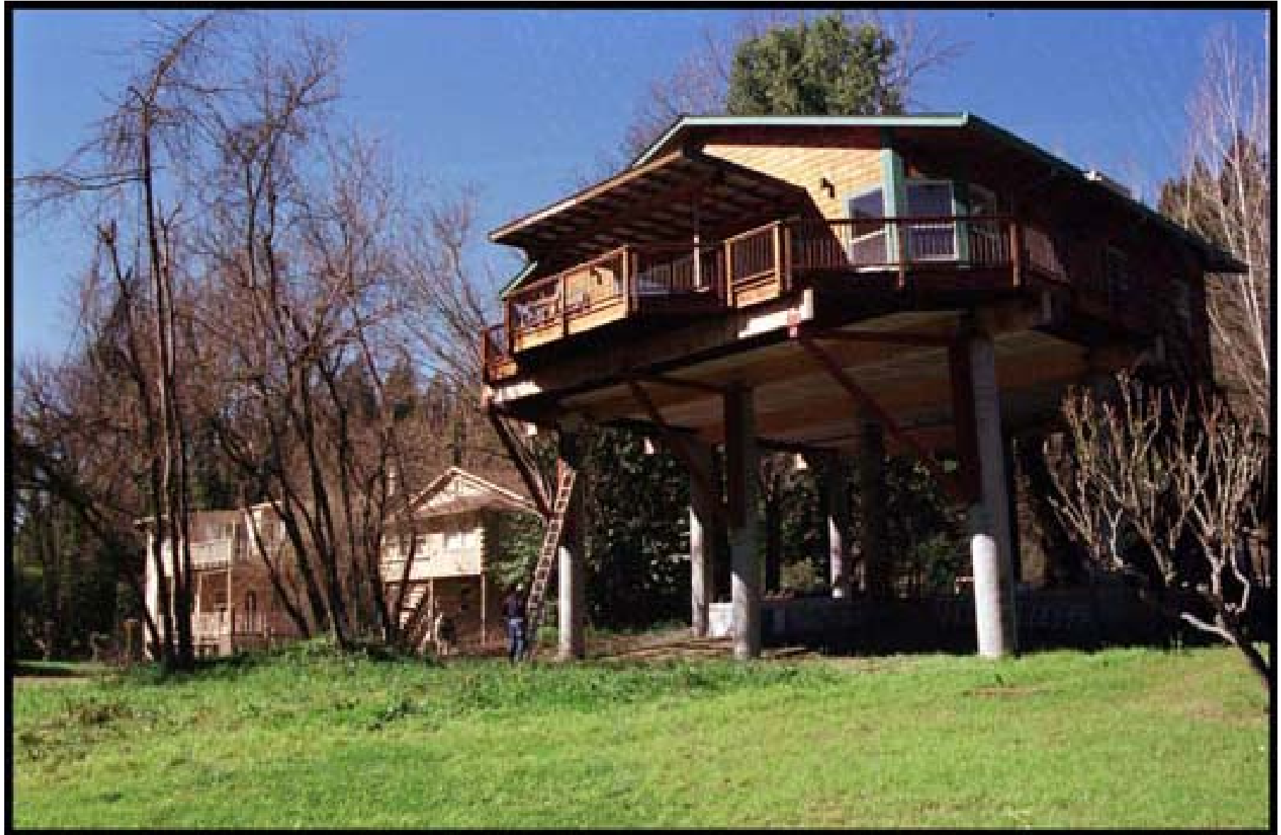
Mitigated home along the Russian River in Guerneville, CA sits 28 feet above neighboring homes. Photo by Greg E. Mathieson/FEMA
