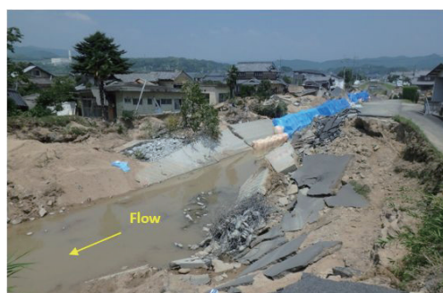
Figure 2 Dike breach along the Suemasa River (Mabi Town, Kurashiki City) 図2 末政川の破堤（倉敷市真備町）
