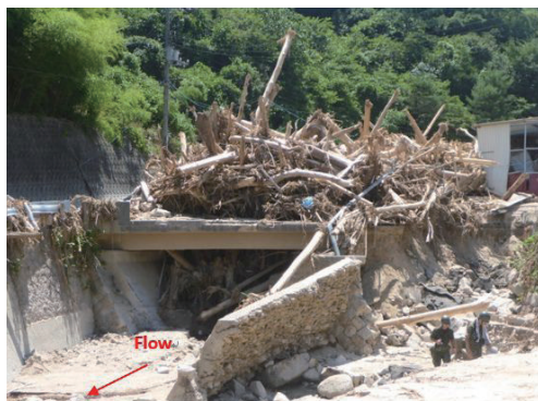
Figure 4 River channel filled with driftwoods at a bridge (Sozu River, Saka Town, Aki-Gun)
