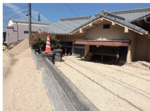
Figure 5 House half-buried with flood-transported sediment (Tenchi River, Saka Town)
