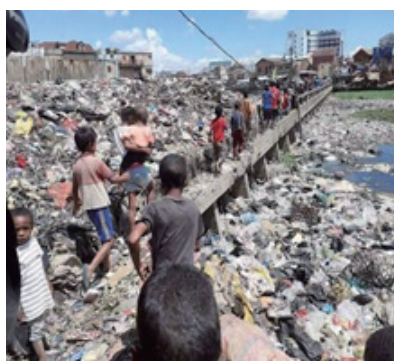
Figure 1. Solid waste blocking drainage canal at bridge crossing, Antananarivo
