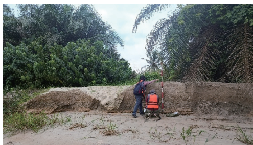
Photo 5 Post-flood survey of riverbank erosion and sediment deposition after rainy-season flooding
