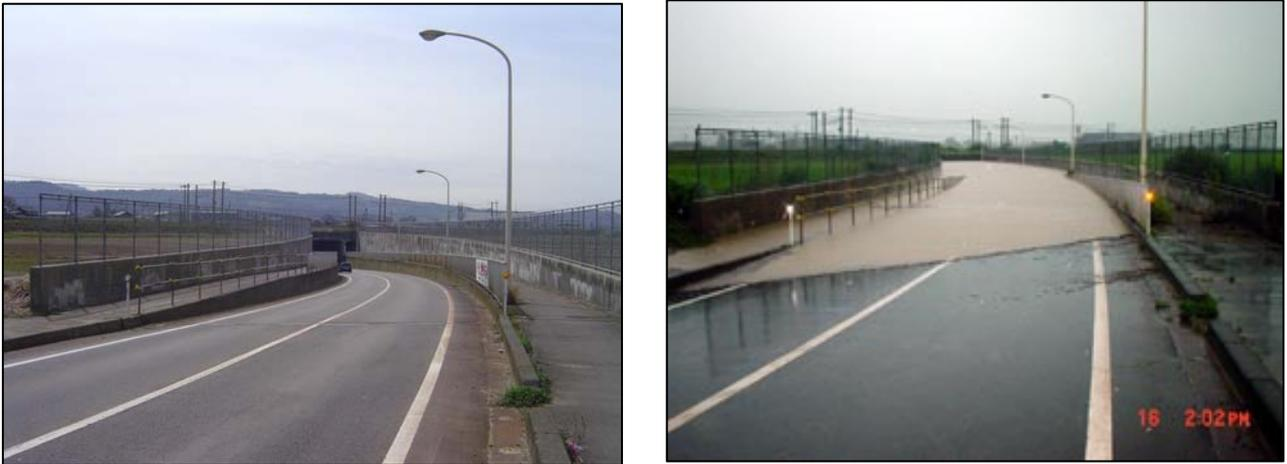
Fig.6 Inundation at an underpass (left – at normal times; right – during flooding) (Sanjo city, Niigata Prefecture)
