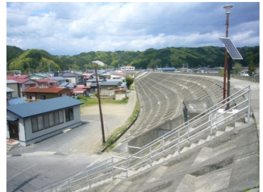
A tsunami embankment in Taro district, Miyako City (height: 10m)
