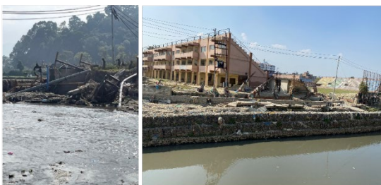
Photo 4-12,13,14,15,16 Damaged infrastructure and houses in the Kathmandu Valley
