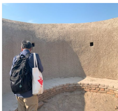
Photo 4-26, 27 The ruins (walls, stupa domes, etc.) are being capped with slurry or mud to protect them from extreme climatic and weather conditions.
