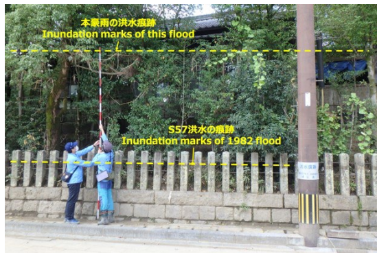
Photo 4-5 Inundation marks at the Aoi Aso Shrine
