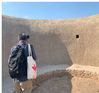
Photo 3-26, 27 The ruins (walls, stupa domes, etc.) are being capped with slurry or mud to protect them from extreme climatic and weather conditions.
