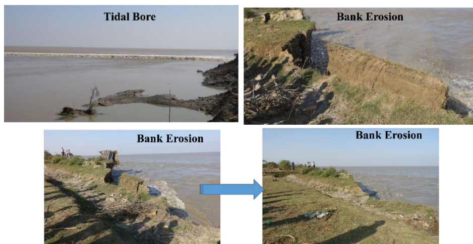
Photo 3-18, 19, 20, 21 Riverbank erosion caused by tidal bores
