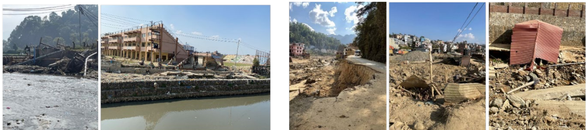
Photo 3-12,13,14,15,16 Damaged infrastructure and houses in the Kathmandu Valley
