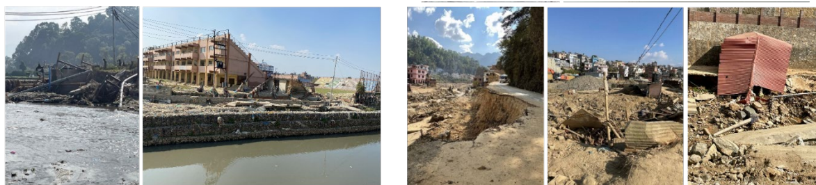
写真 3-12,13,14,15,16 Damaged infrastructure and houses in the Kathmandu Valley
