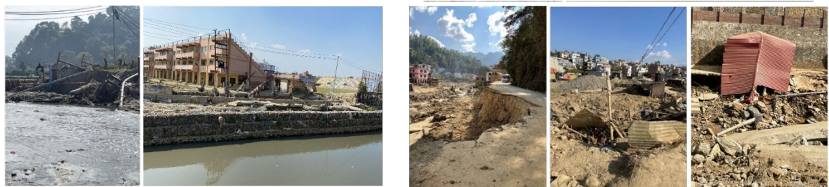
写真 6,7 Damaged infrastructure and houses in the Kathmandu Valley
