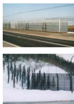
図-5 防雪柵の端部対策例
